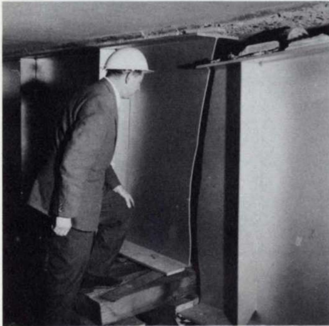
Figs. 1a and 1b King's Bridge, Melbourne. Welded girder bridge of B.S. 968 (1941) steel Collapsed 1962
