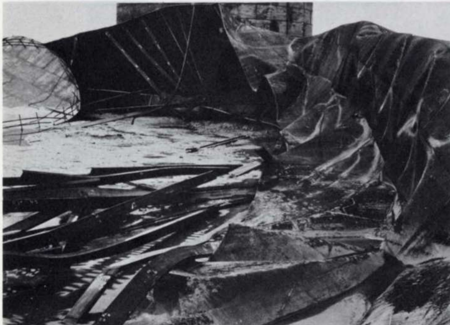
Fig. 1c Petrol storage tank at Fawley of welded B.S.15 steel Collapsed during pressure tests, 1952
