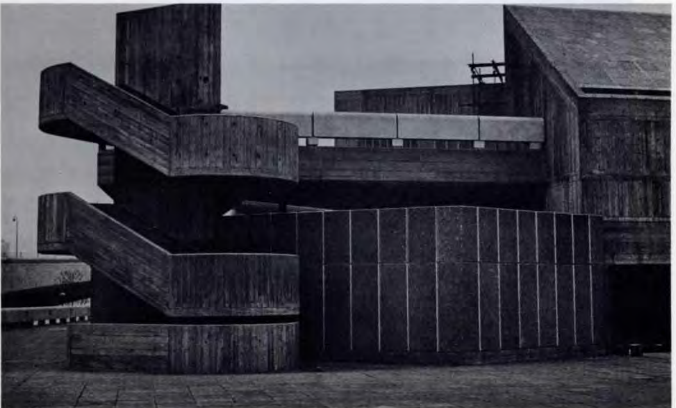
Fig. 15 Typical external staircase.
