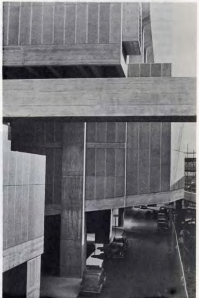
Fig.10 A view of the Purcell Room cantilever. Note the plant room above and its supporting structure. Prestressed concrete footbridge connecting high pedestrian levels in the foreground.
