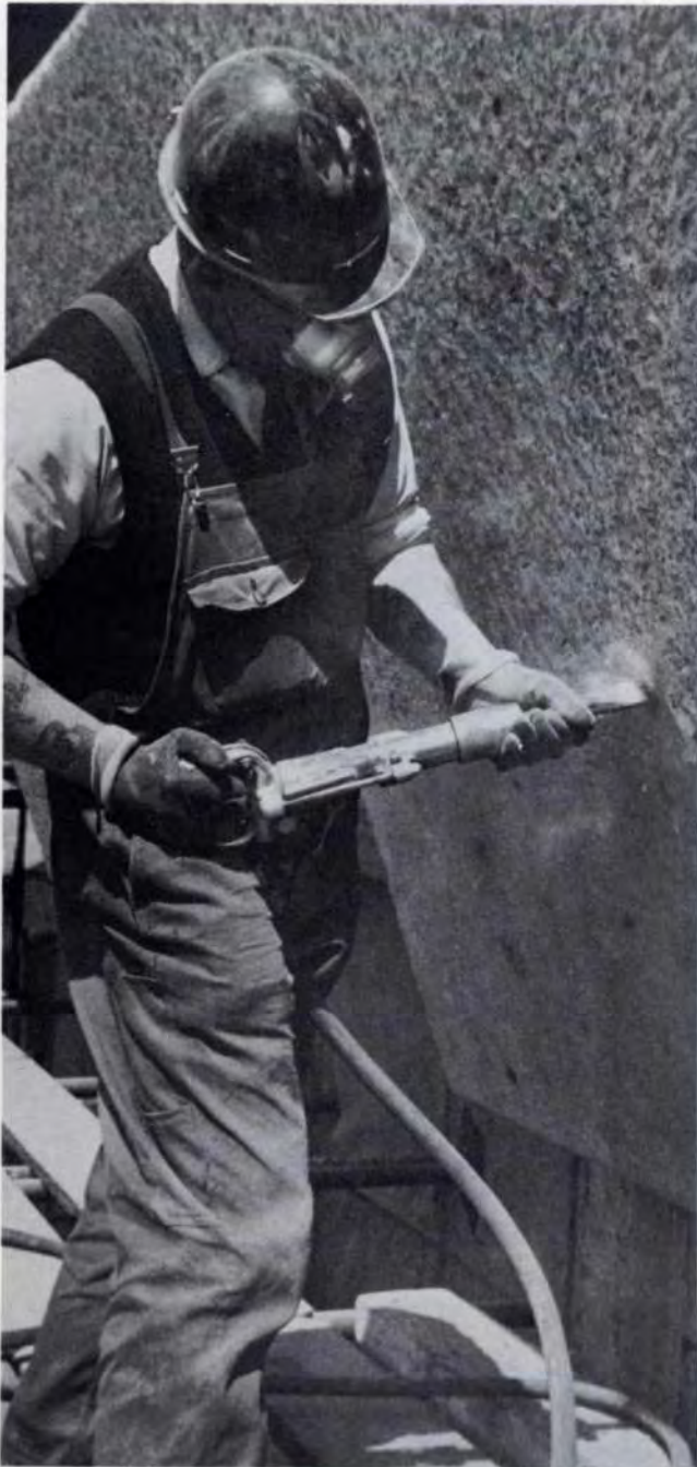
Fig. 12 Block 6. Pick-hammering with a chisel bit
