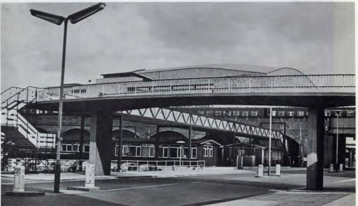
Fig. 4 Upstream Belvedere Road footbridge and temporary walkway link
