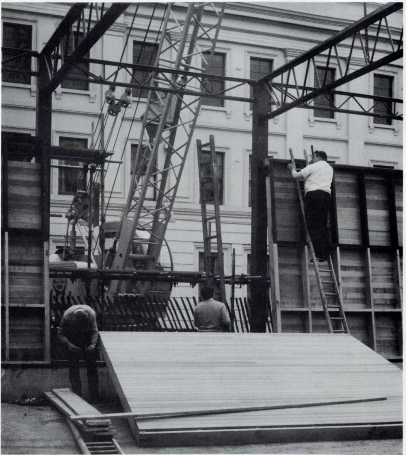
Fig. 7 Erection of wall panels in Riding School Photo: Axel Poignant
