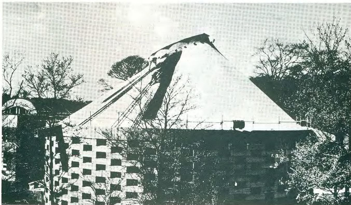
View of completed concrete shell (photo: E. Mark)
