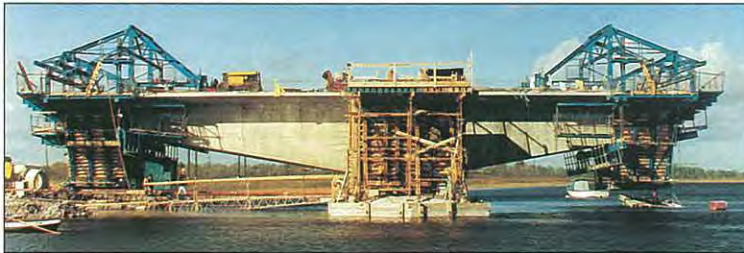
10. & 11. Cantilevering in progress.
