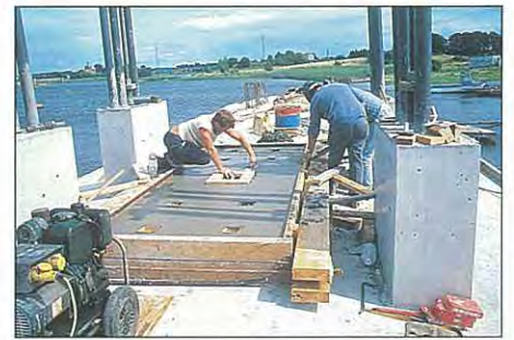
9. Installation of bearing plinth, temporary props.
